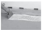
Stir glue thoroughly before use. Apply with notched applicator, coverage approx. 800-1000 g/m<sup>2</sup>. Insert the flooring boards within 15 minutes. Start with the tongue side parallel to the wall in the case of Tongue and Groove plus.
